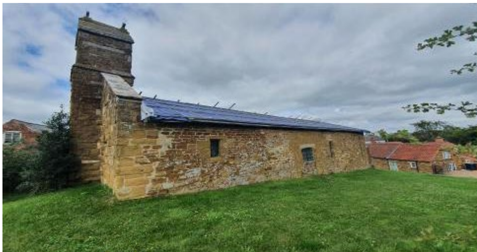
Figure 6: St Leonards has an easily accessible roof
