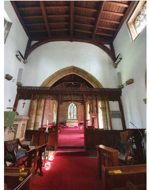
Figure 8: The chancel already has a partition and separate heat source.
