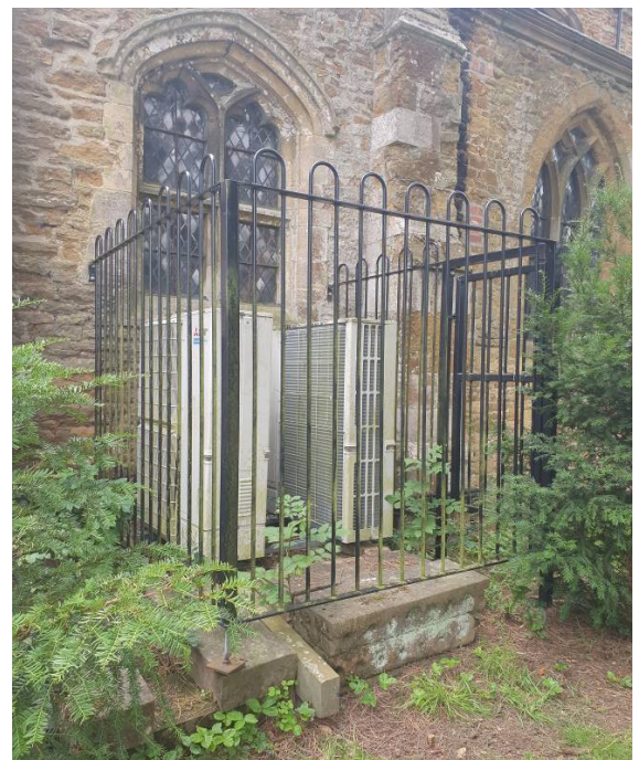
Figure 4: Fan Unit at St Egelwins
