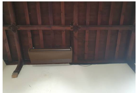
Figure 3: Air Blower at St Egelwins
