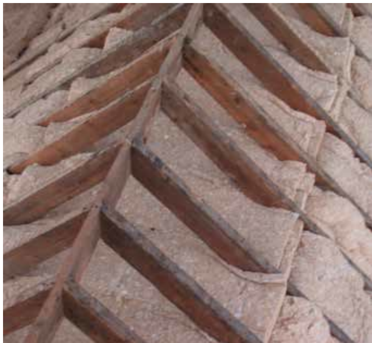
Figure 2: between rafter insulation. Image courtesy Historic England
