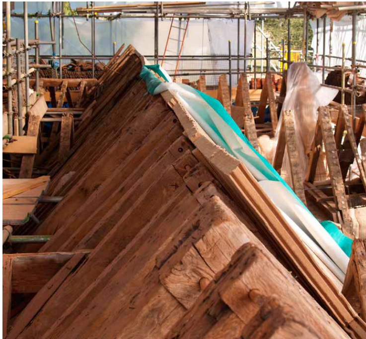
Figure 1: Above rafter insulation using wood fibre board. Image courtesy Historic England
