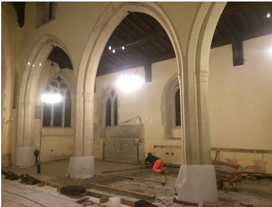
Figure 5: SubLime floor installation at Chrishall Church near Duxford. image source limecrete.co.uk
