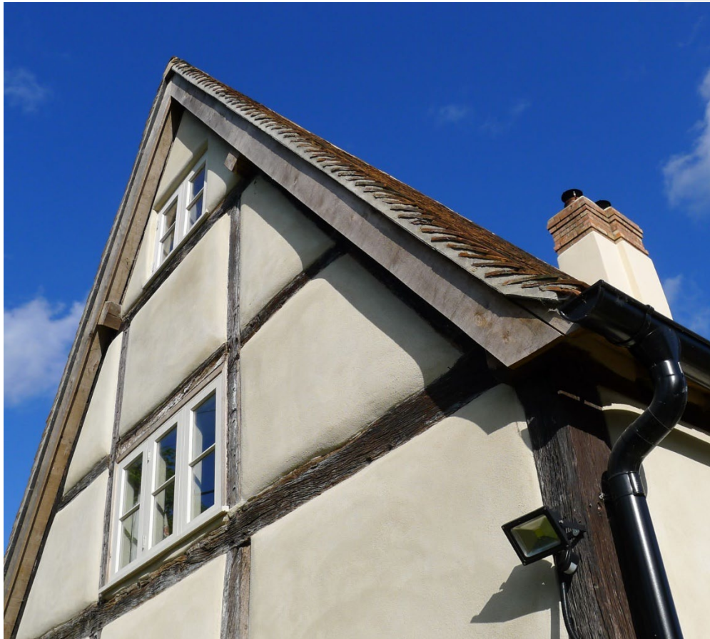
Figure 4: wall insulation feathered to reveal historical details
