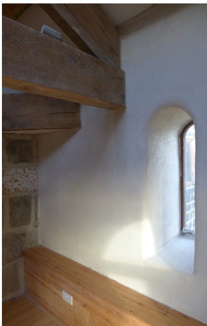
Figure 3: internal hempcrete solid wall insulation (UKhempcrete.com)
