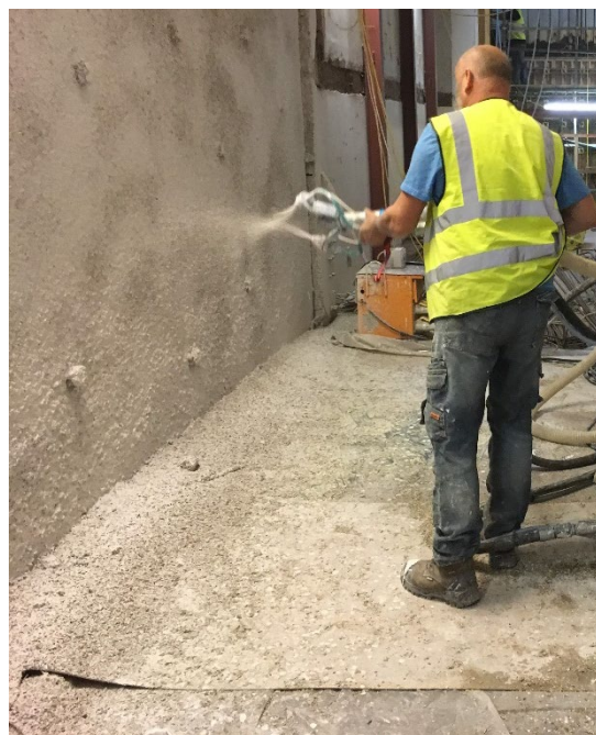
Figure 3: internal hempcrete solid wall insulation (UKhempcrete.com)
