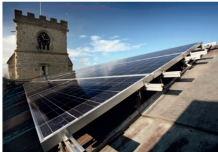
Figure 9: Photovoltaic panels on the roof of the nave at Wing All Saints, Buckinghamshire (Photo: Martin Findlay)
