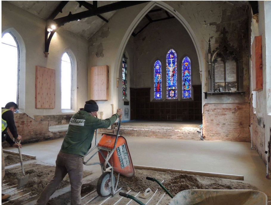
Figure 6: SubLime floor installation at St Margaret's Church, Ward End, Birmingham. Image source limecrete.co.uk
