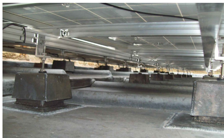
Figure 8: PV mounting on lead roof; mounting system shown from below panels (image source Historic England)
